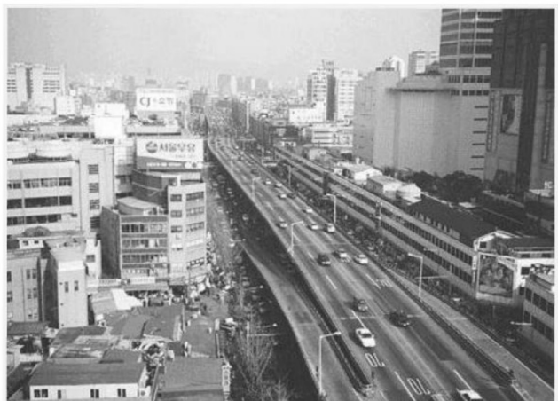
After the construction of the overpass
